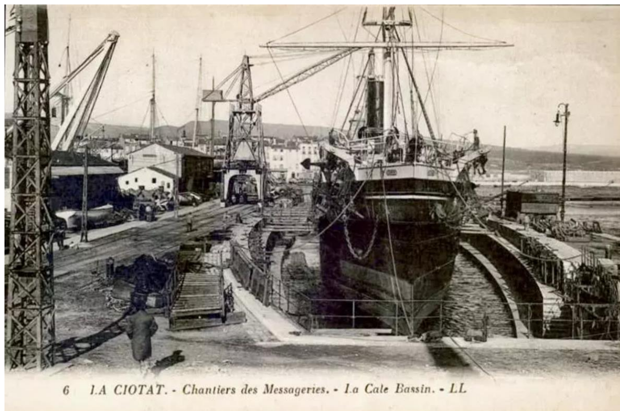
Image 8.1. The shipyard of Messageries Maritimes , the dry dock with its rolling crane in La Ciotat.
