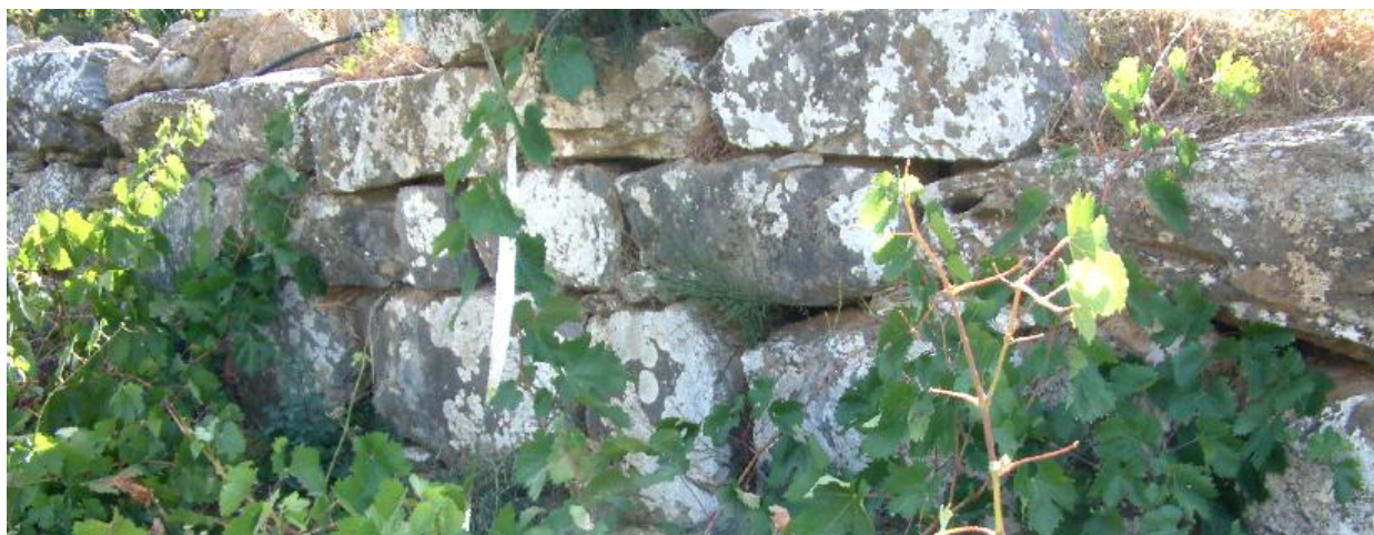
Figure 26: Nearly isodomic big block masonry in retaining wall at Avgo, Kavousi.
