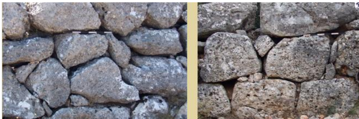
Figure 25: Masonry differences oncolithic PP – Cretan Cyclopean LM III. Left: “Cross-braced” Minoan (Site 99A, N wall). Right: “Isodomic” LMIII (and later) ruin at Kroustas Perdikolakkas (unpublished).
