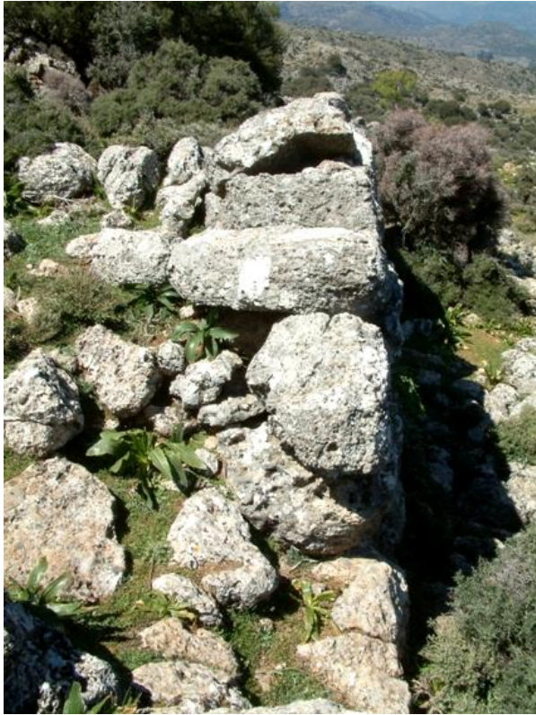
Figure 4: Site 100. Dwelling ruin, E wall seen from S, with diatoni (wall width: 0,8m, height: 2,3m)
