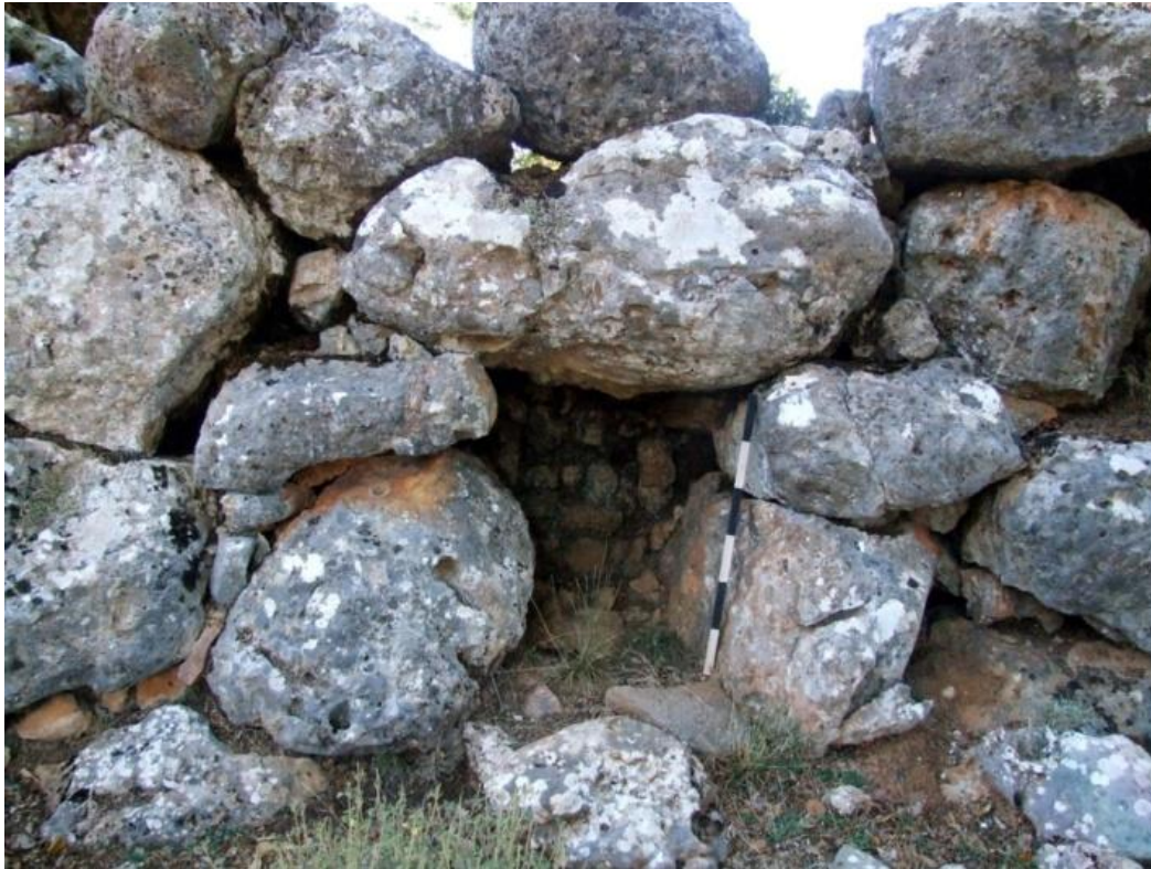
Figure 16: Site 18. Dwelling ruin from below the SE (downslope) ruin wall. Opening probably for drainage.
