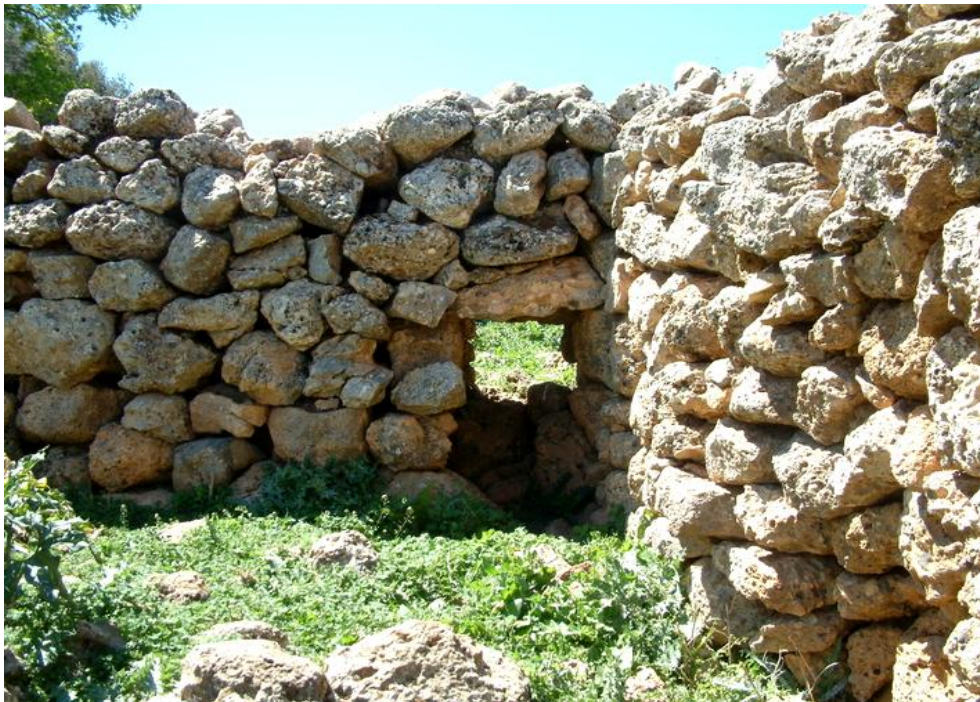
Figure 18: Next to Site 100. Recent mandra outside, downslope side with waste disposal /drainage opening.
