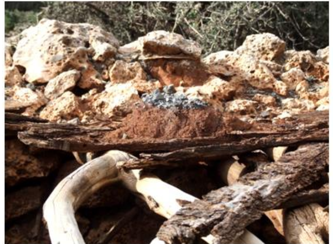
Figure 13: Tsivi South. Two varieties of roofs, slightly inclined for water runoff. Cypress timber and stone slabs positioned like tiles (left) (1200 masl); timber from various trees bark covered, red “domatochoma”, grey gravel (for easy drainage) and stabilising rocks (right).
