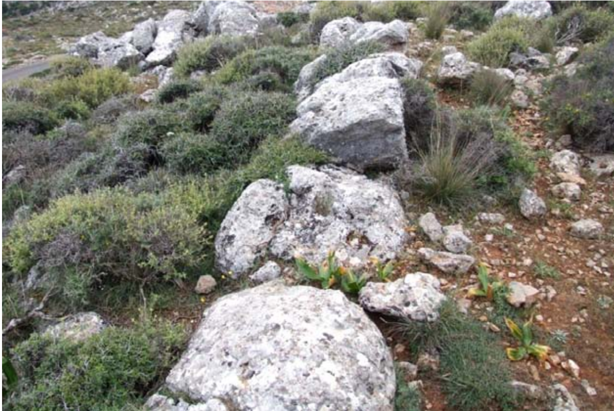
Figure 11: Site 44C. SE wall of dwelling ruin from NE. Type 2.B.3 - Single row double faced
