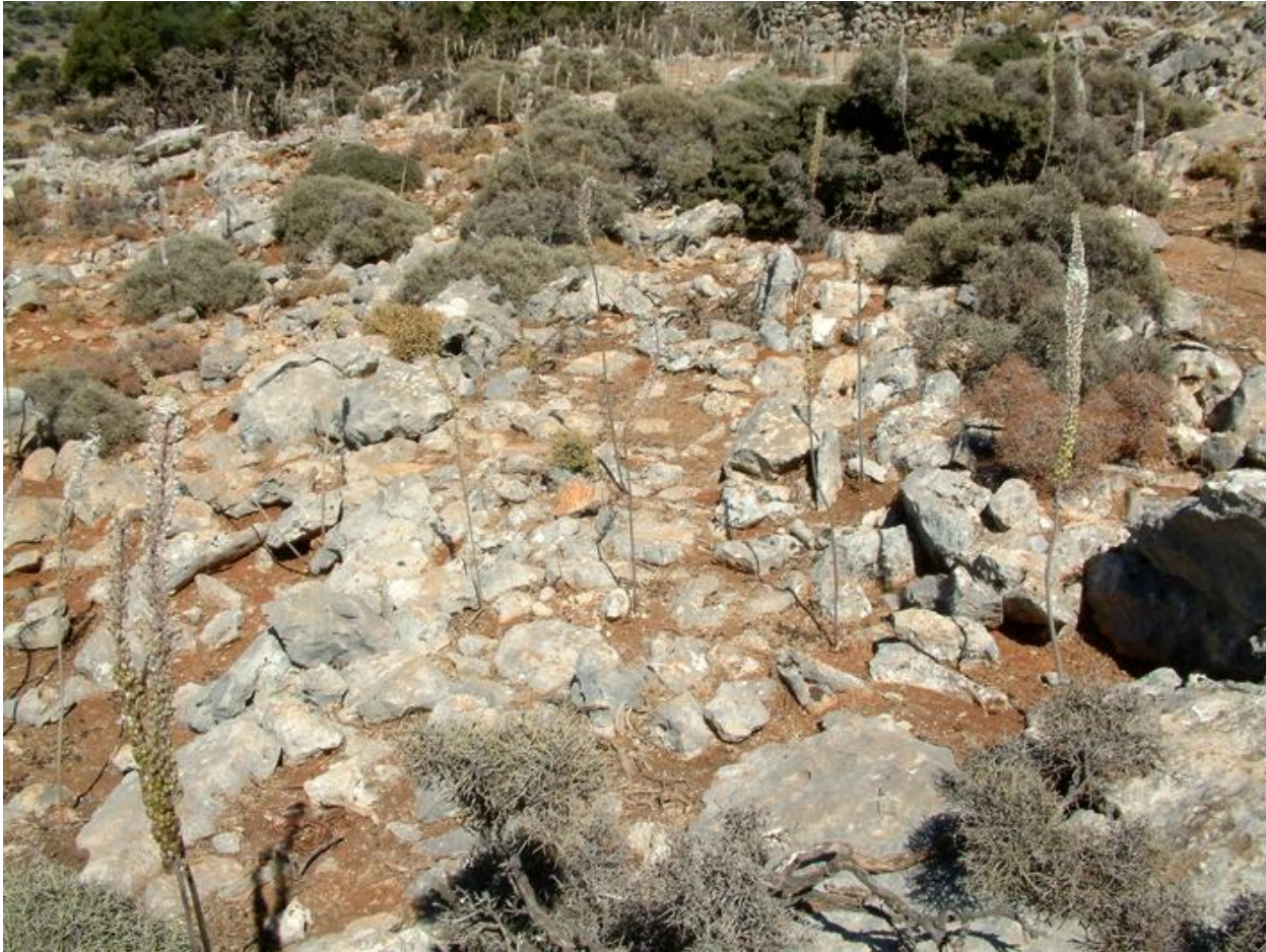
Figure 17: Road type 2 (1,2 m broad) SW of Site 54. Rubble paving raises the level of the road above the surrounding terrain.
