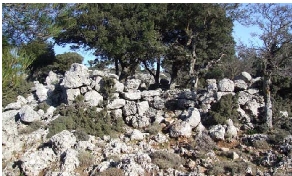
Figure 6: Site KA10. Building remains (standing up to 2,2 m). W wall from W
