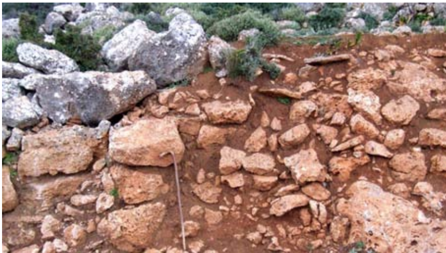
Figure 3: Site 44D. The bulldozer-cleaned NE corner (above stick, length 90 cm). The stone slabs on the uphill outside, obviously intended for levelling the ground, are covered by only 20 cm of colluvium, trapped between ruin and slope
