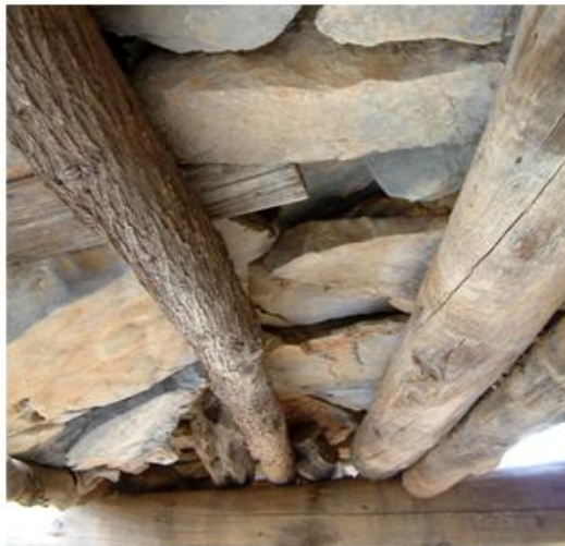
Figure 13: Tsivi South. Two varieties of roofs, slightly inclined for water runoff. Cypress timber and stone slabs positioned like tiles (left) (1200 masl); timber from various trees bark covered, red “domatochoma”, grey gravel (for easy drainage) and stabilising rocks (right).
