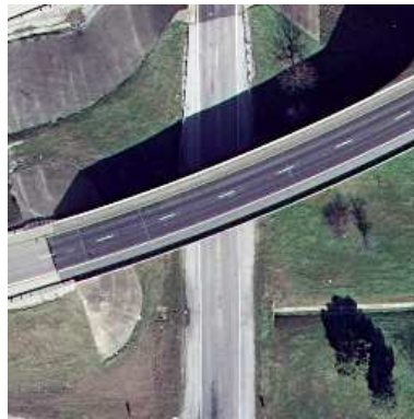
(b) bare soil , grass , pavement , trees , cars
