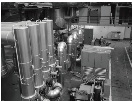
Figure 6.2.1: Representative image of the machine hall, where the EuRoC micro aerial vehicle dataset was collected.
